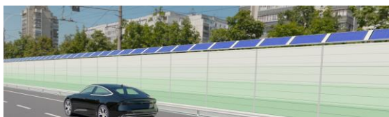
Figure 3: Illustration of an upgraded noise barrier, referred to as “PVNB (Upgrade)”. The modules are installed on the ridge of existing barriers. Copyright: Fraunhofer ISE.
